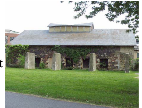
(Stone front of the original mill at Fibermark Inc.)
